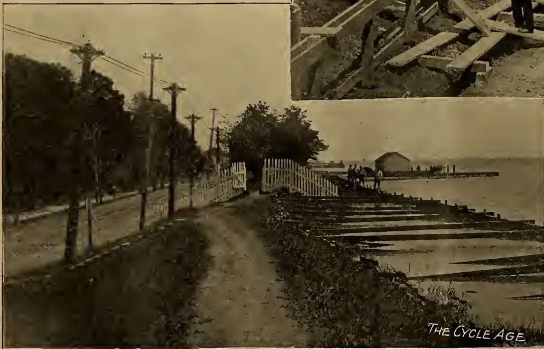
LEVEE FRONT AT JACKSON BARRACKS
